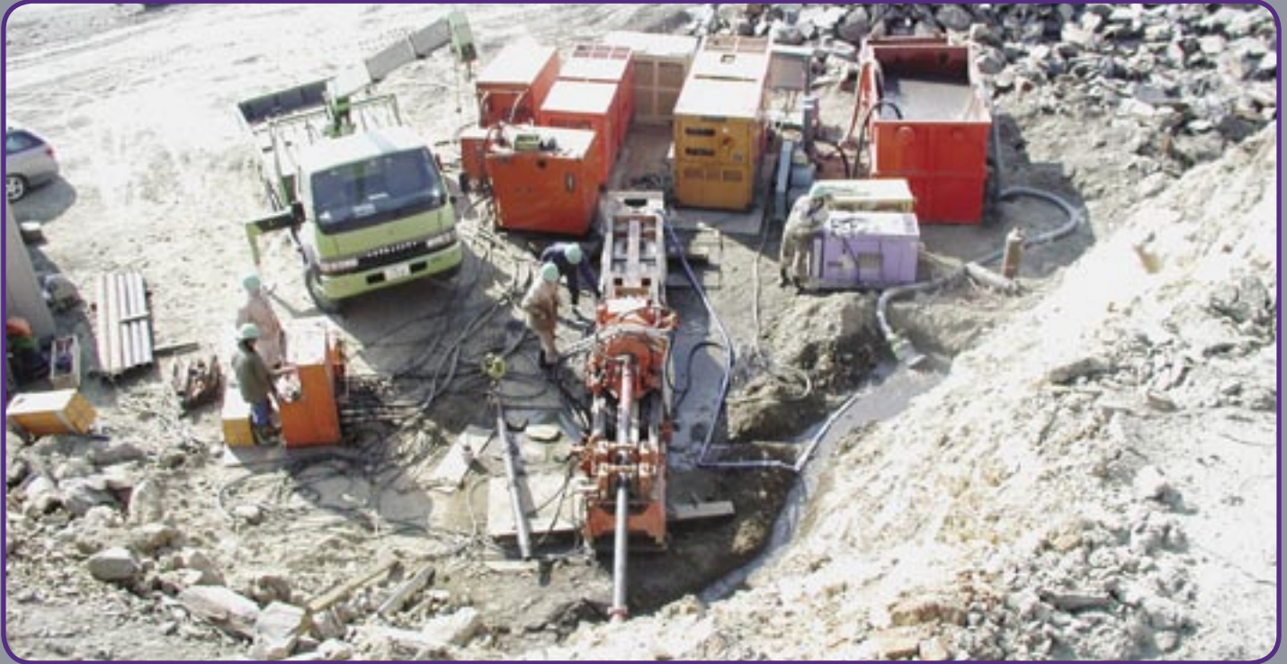
■ Installing horizontal drains to improve slope stability of a mountainside.
