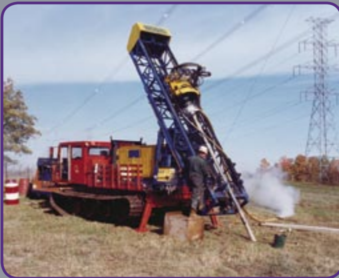
■ Angle drilling to install hydro-electric transmission tower guy wire anchors.
