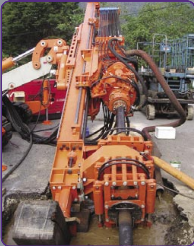
■ Installing tie-back anchors for a retaining wall.
