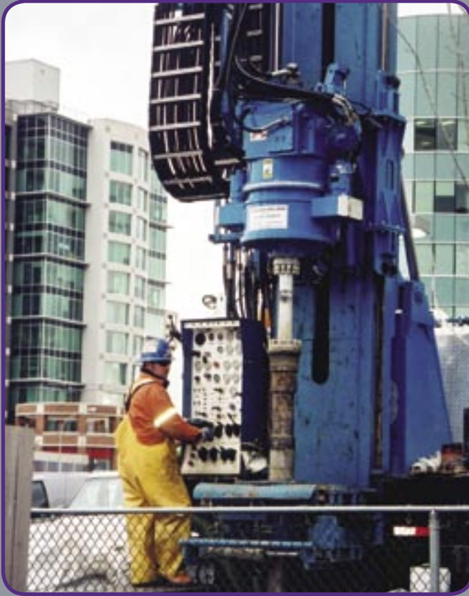
■ Drilling for geotechnical investigation of a high rise residential building site.
